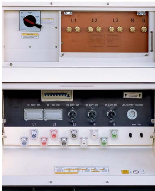
Lug and camlock connections
